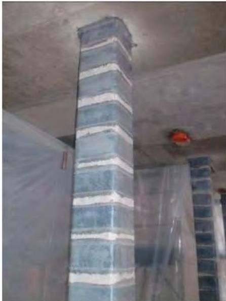
carbon fibres wrapping to increase the shear strength in a column
