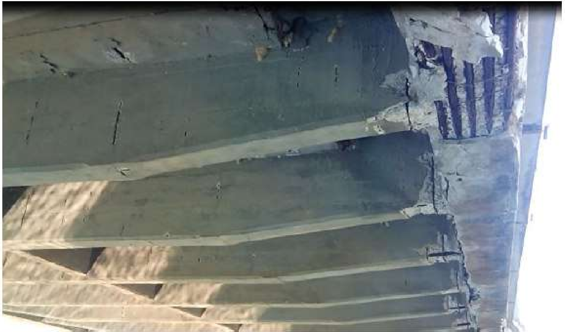
Figure 2 – Cross beam and thrust beam/Traversi e trave reggispinta
